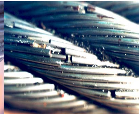
Fatigue broken wire
